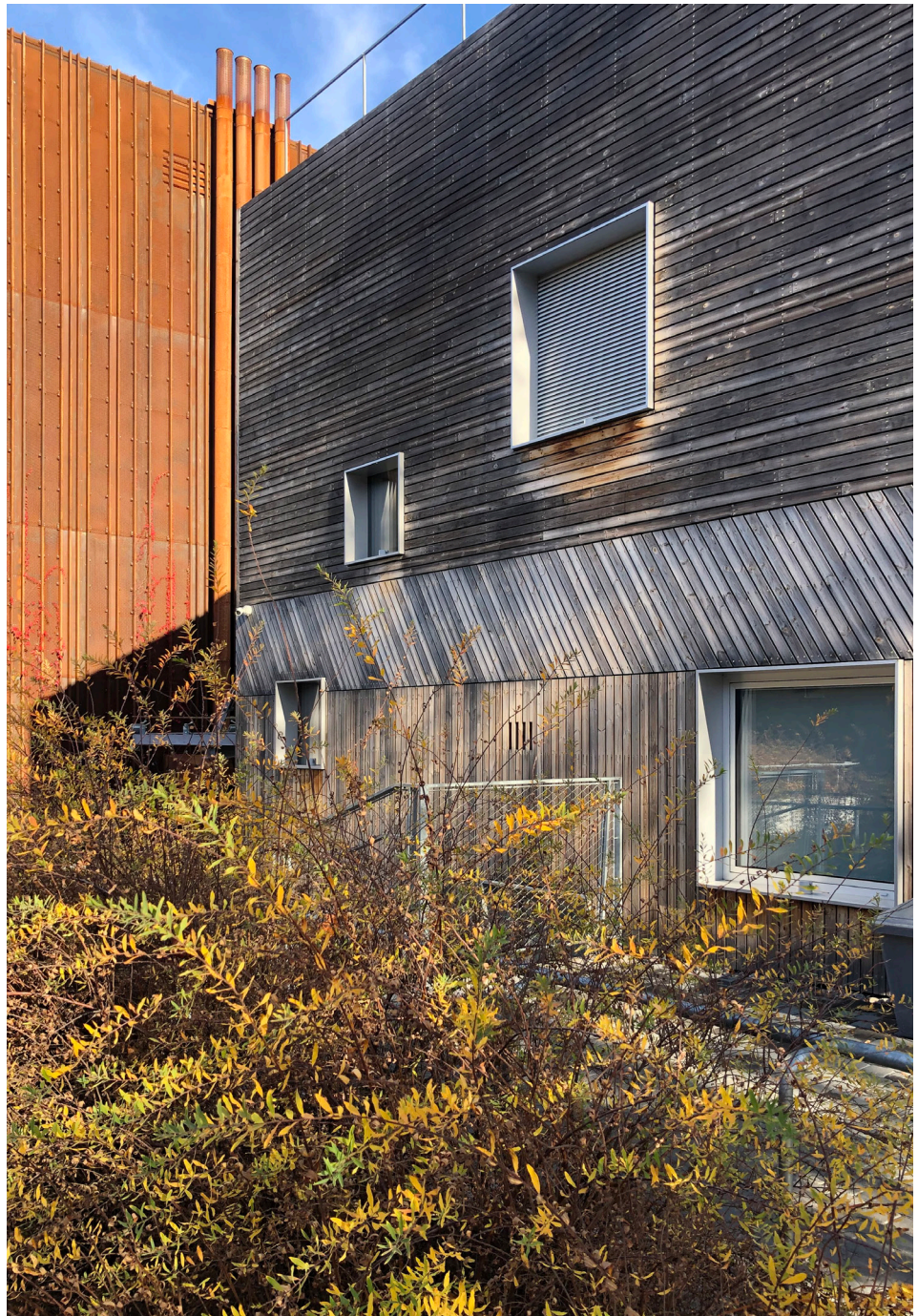
Pasaka Cinema Boutique in Paupys // Vilnius, 2019-2020 // Profiles: Batten 42x68 (façade and roof), batten 42x92 (terrace and benches) // Not coated // Architect: Audrius Ambrasas Architects // Photo: Joana Suslavičiūtė
