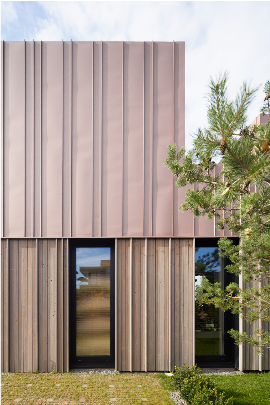
Residential building in Gulbinai // Vilnius, 2020 // Profiles: Rombas (20x92), Mykolas (26x68) // Coating: Teknos 1707 // Architects: 2XJ // Photos: Norbert Tukaj
