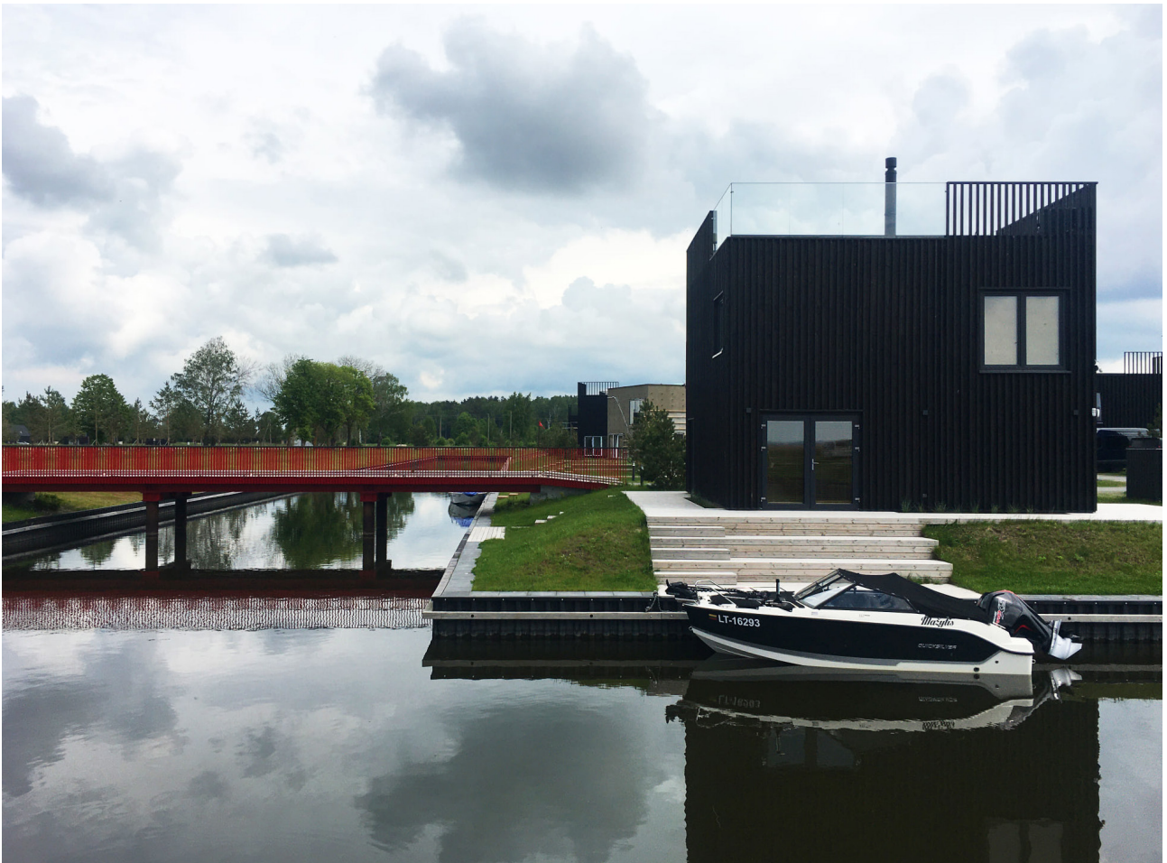
DO ARCHITECTS, Svencelės salos // Profiles: Mykolas (19x92, 19x117, 26x68, 42x92, 42x140) coated in black Tikukurila Wood Stain 5089, terrace Mykolas (26x117) not coated // Architects: DO ARCHITECTS, Karresen Brand (master plan) // Photos: DO ARCHITECTS, Svencelės salos
