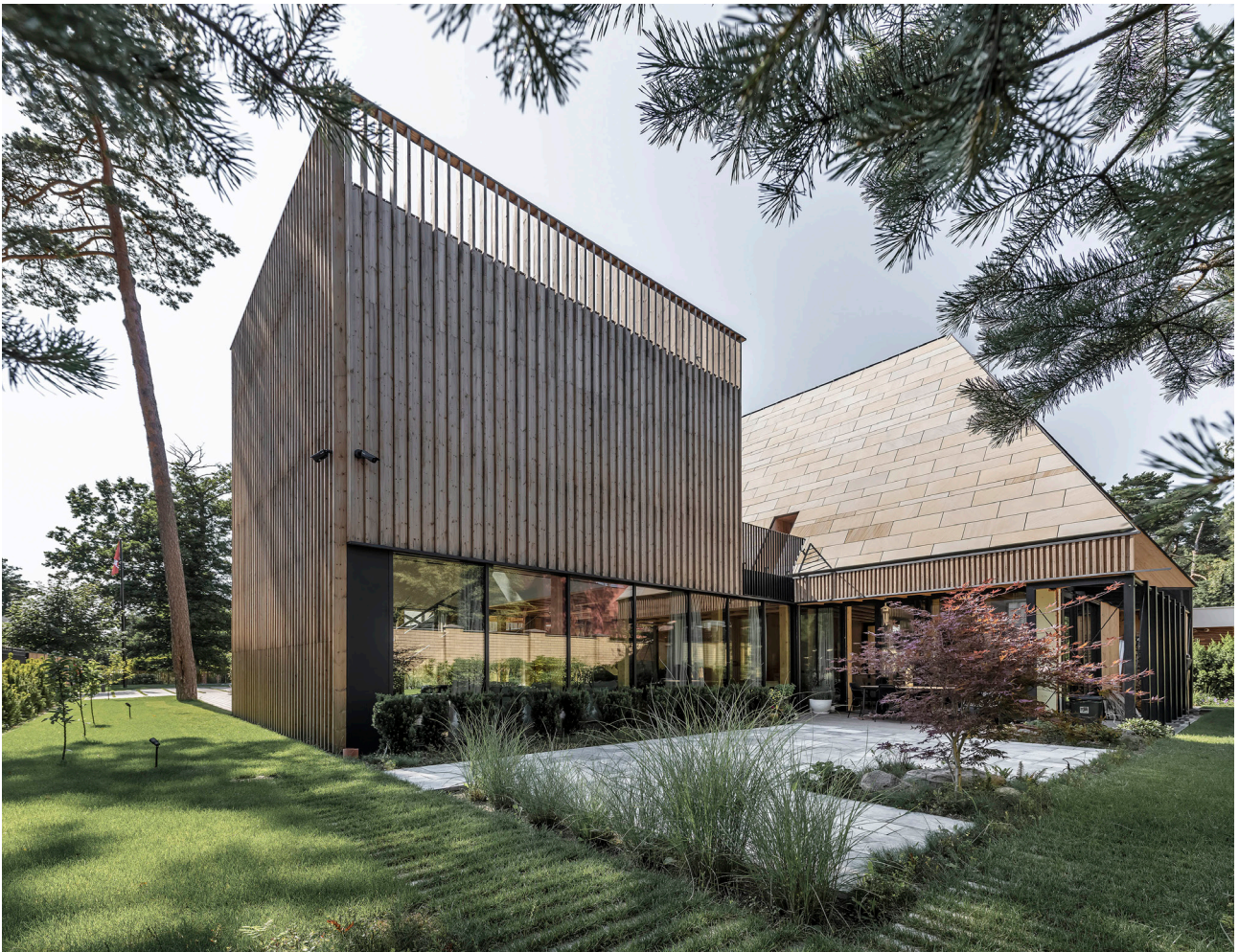
Family villa in Giruliai // Giruliai, 2019 // Profiles: Battens (42x42, 42x68, 42x92) coated in clear oil, terrace Jonas (26x117) // Architects: DO ARCHITECTS (Andr  Baldi iut , Algimantas Neni kis, Julija  iapait  – Jurevi ien , Kasparas  iliukas) // Photos: Laimonas Ci unys, DO ARCHITECTS
