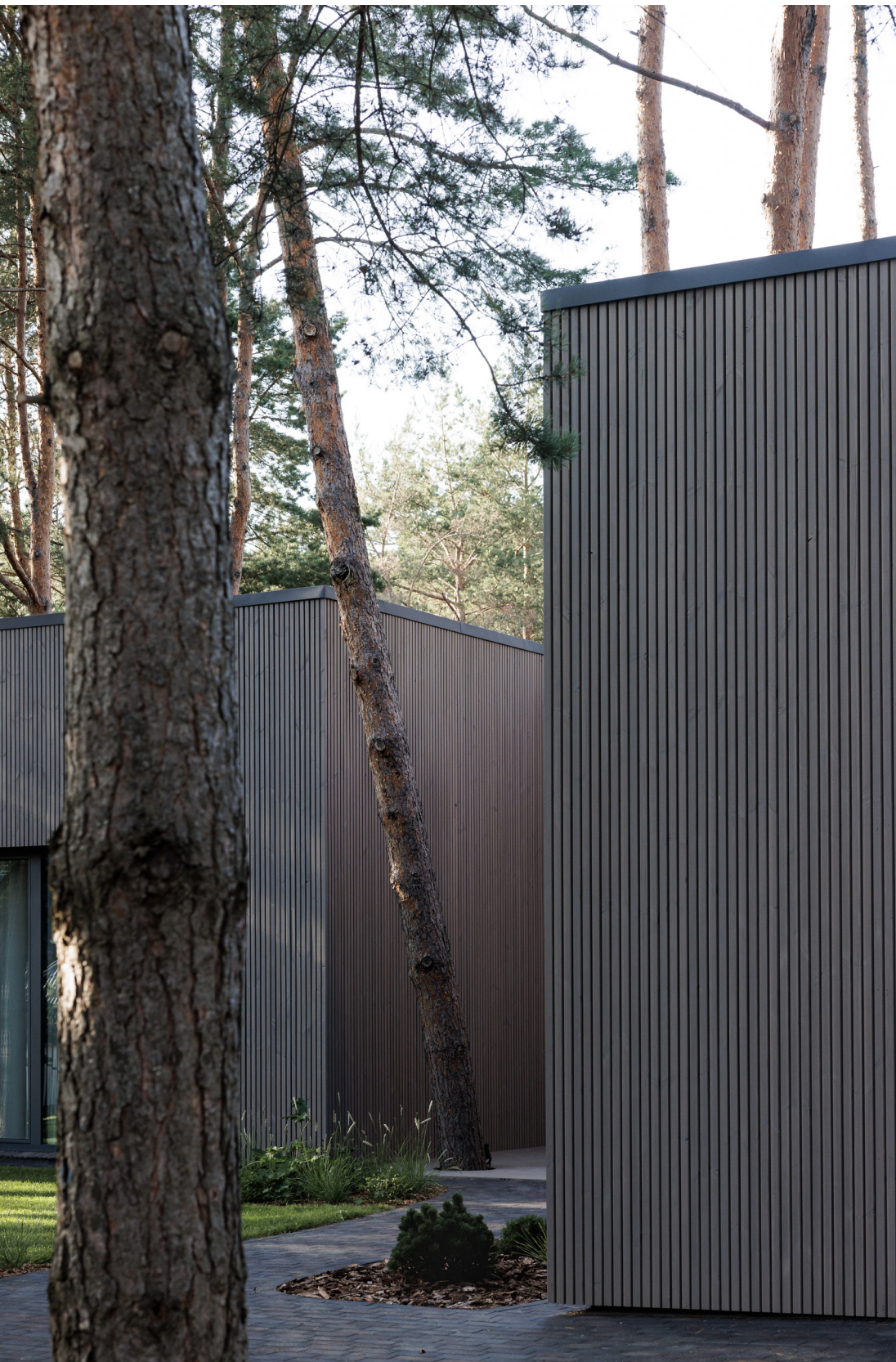
Private residential building // Kaunas, 2023 // Profiles: Mykolas 26x117 and Grète 32x142 // Coating: TK WS 5147, not textured // Architects: Nebrau Architecture // Photo: Norbert Tukaj
